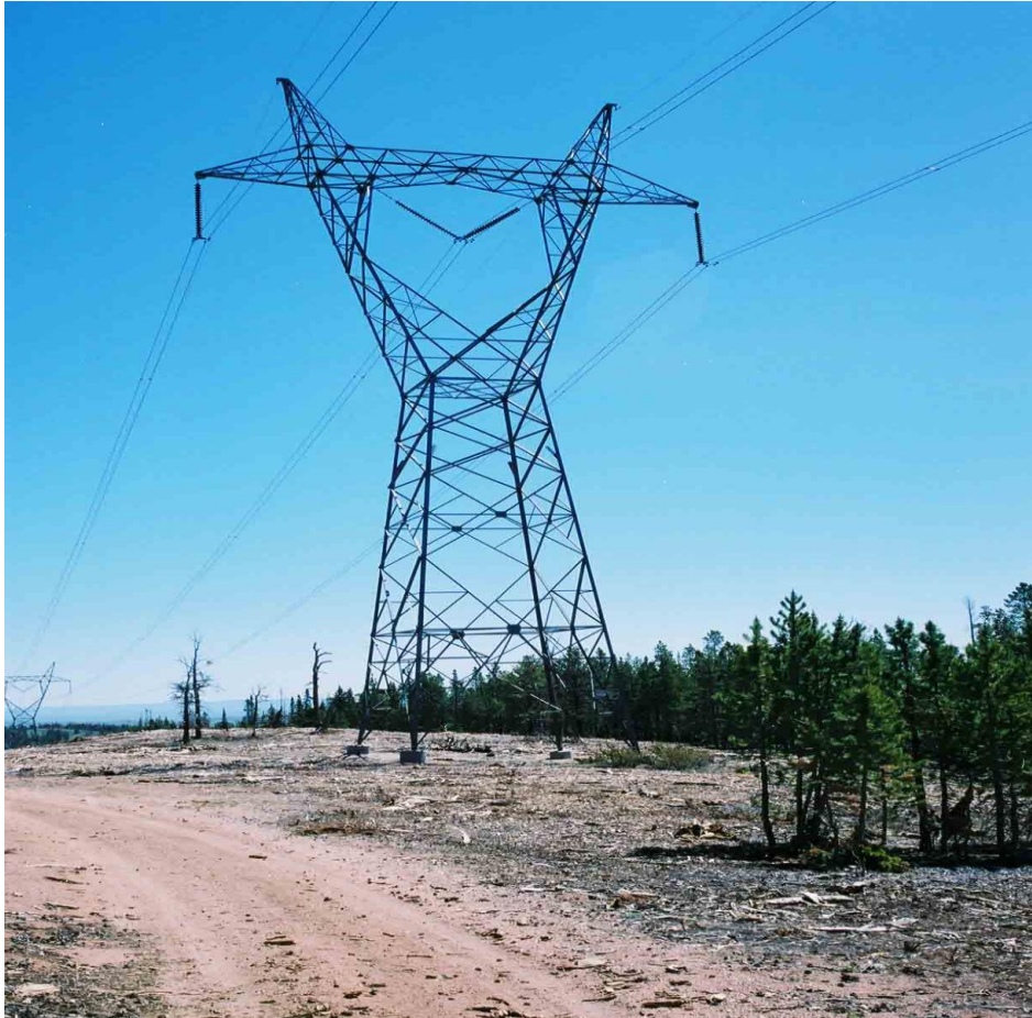
Figure 8-8: Vegetation management through chipping.
