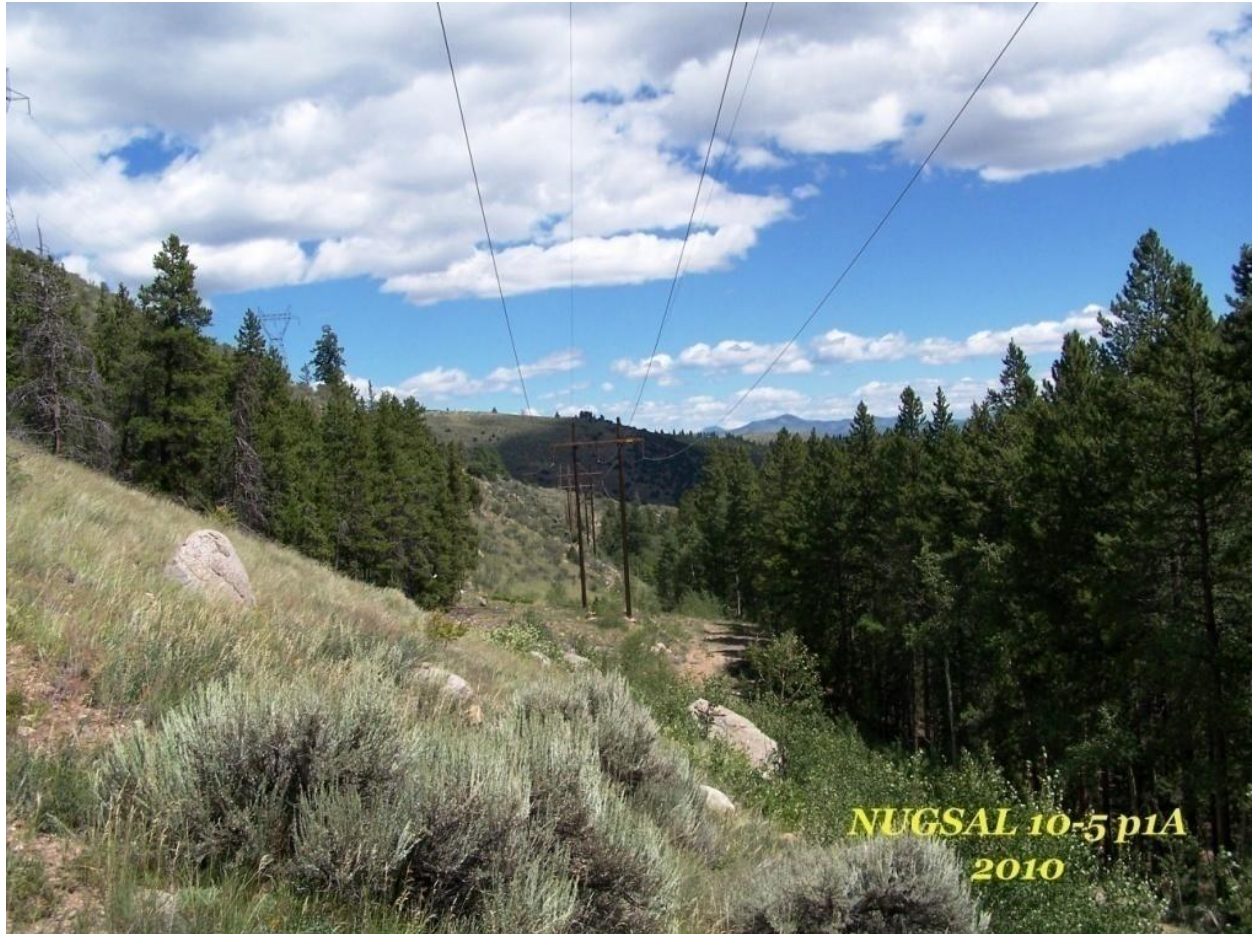
Photo 2-14. The condition of this ROW is generally acceptable and relatively stable, but will require monitoring to ensure that the need for treatment can be identified and implemented. Note the low level of aspen re-growth in the lower right corner, which has emerged and must be closely monitored.
