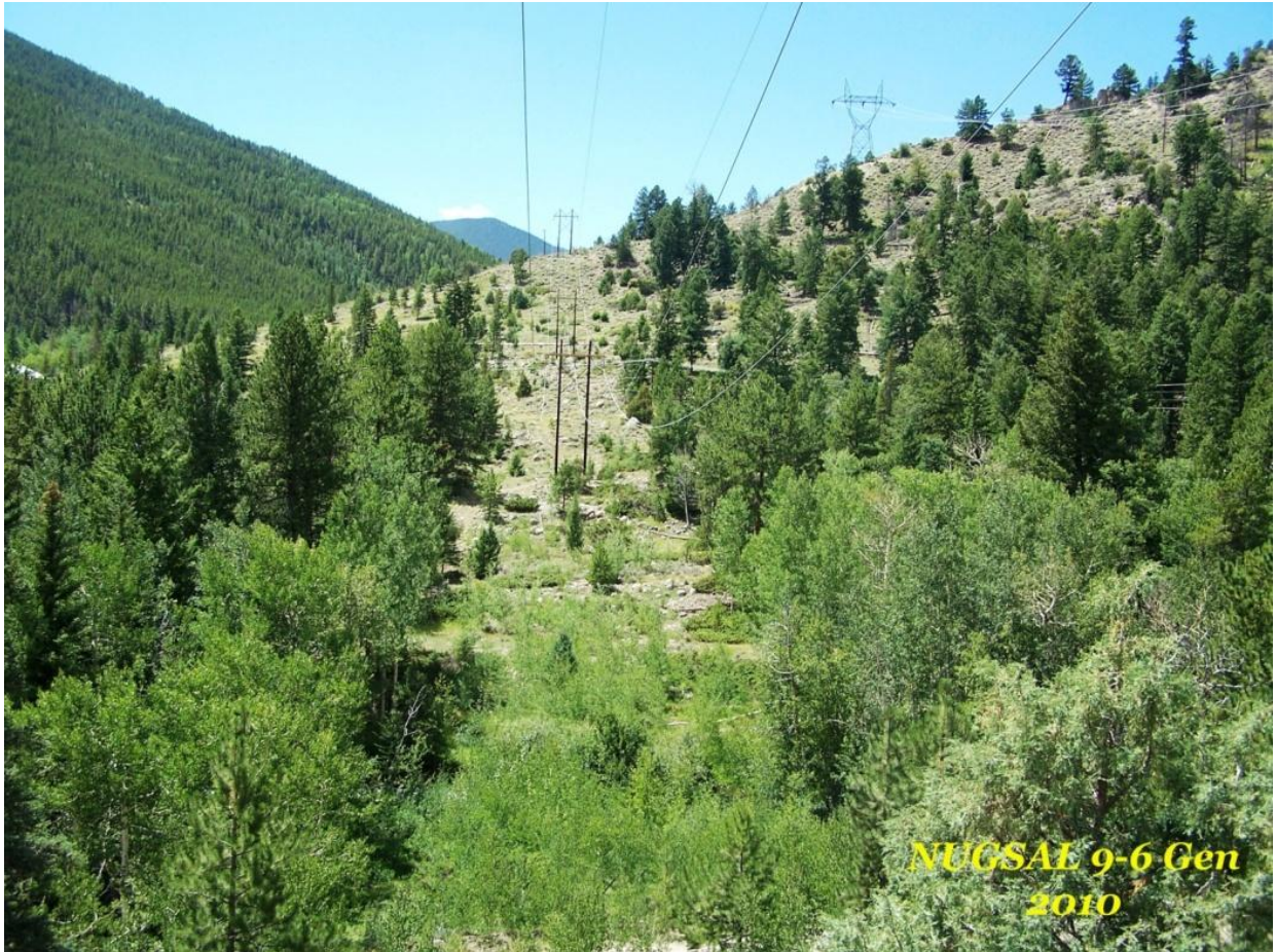
Photo 2-9. In the foreground, aspen, a fast-growing incompatible species, would need to be treated and then maintained in a low-growth condition. In the background, slower-growing evergreen species have not become a problem since the line was constructed; this is typical of Category 5 conditions. The photo also illustrates that there can be different types of vegetation conditions in a small section, and underscores the need for routine monitoring of ROWs.
