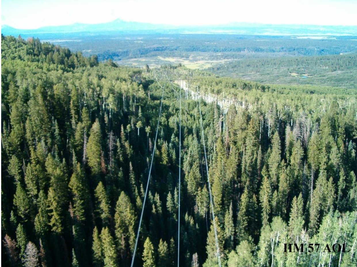
Photo 2-4. Incompatible conifer and aspen vegetation that would require initial treatment to establish a low-growth condition, which Western would then maintain. In the middle of the photo, note how the aspen in the ROW have vigorously re-grown after numerous treatments.
