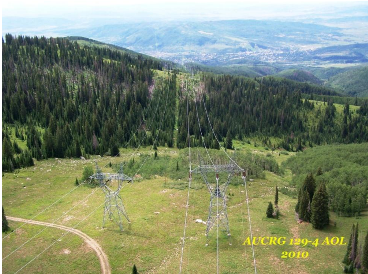
Photo 2-2. The transmission line spans vegetation in a drainage that is unlikely to present a risk to the transmission line, and would not require intensive treatment. Aspen patch immediately behind the foreground towers would require intermittent treatment. Conifers near and in the bottom of the drainage area would not.
