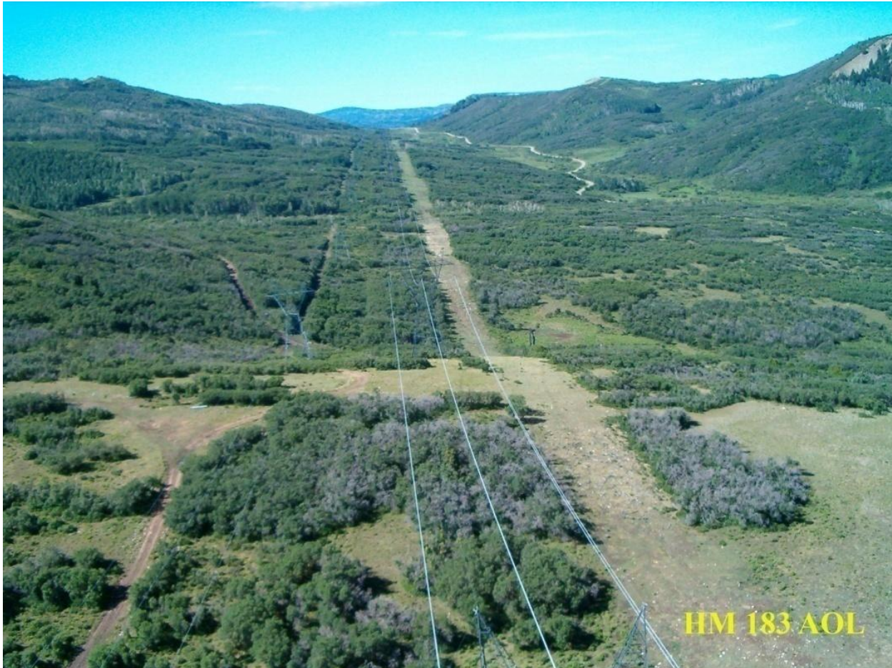
Photo 2-17. There are two parallel transmission lines and a pipeline in this utility corridor. This dense vegetation around structures and under the conductors could present a fuel problem. Note the dead vegetation under the transmission line in the foreground.
