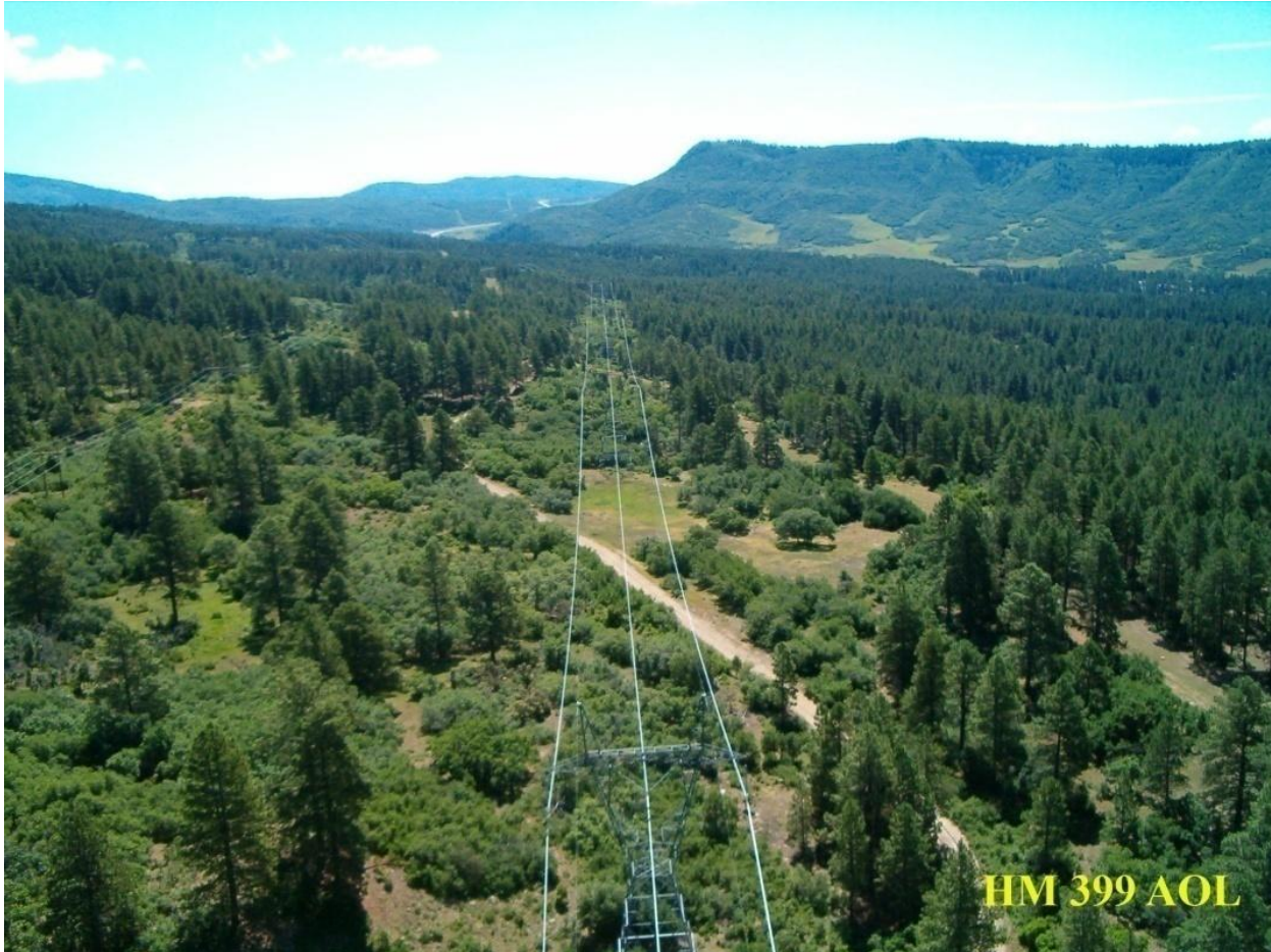
Photo 2-16. Western would monitor potential fuel loading under the lines and near the structures, and schedule treatment as needed.
