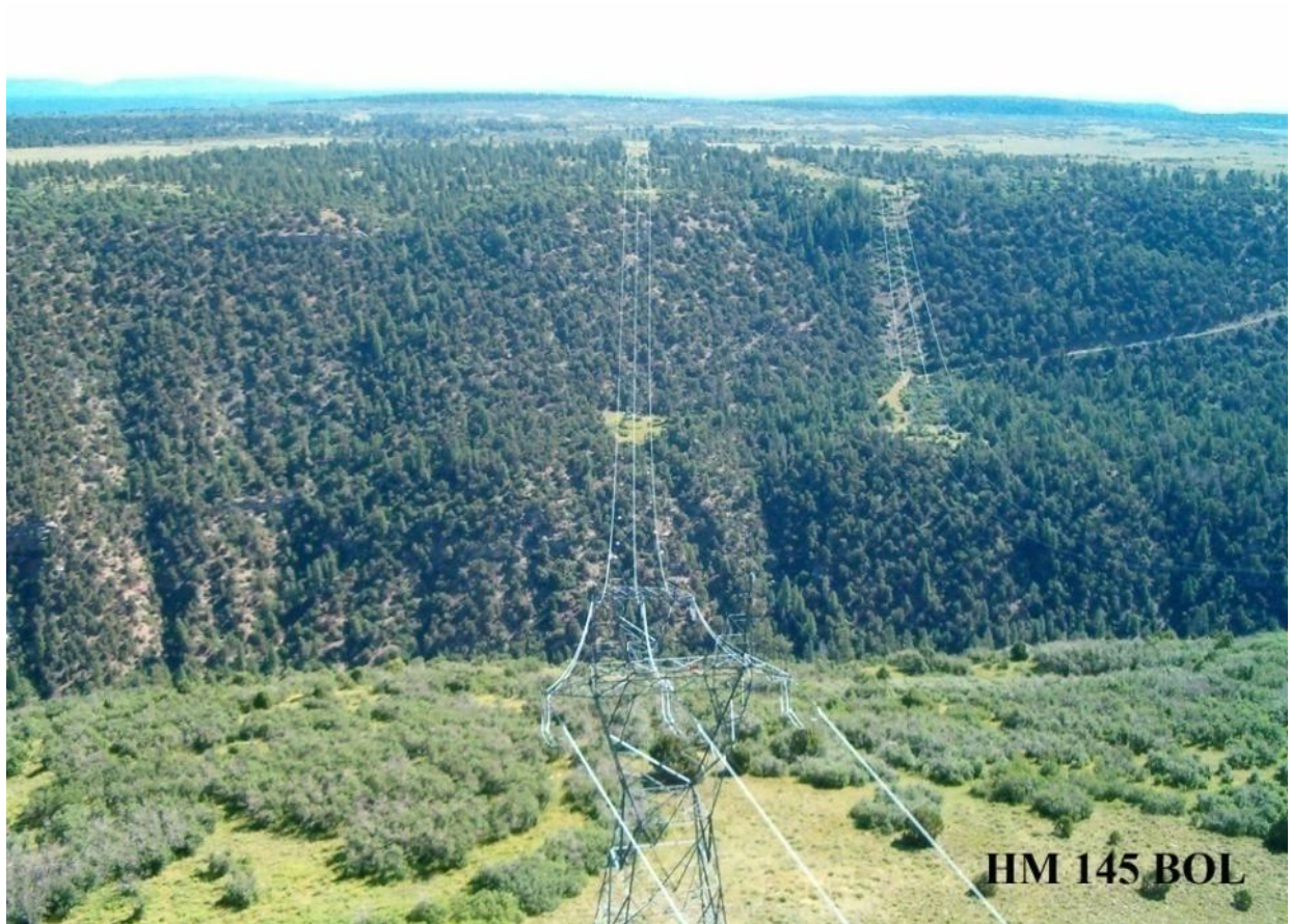
Photo 2-3. Transmission line spans vegetation that would not require treatment. However, note that at the structure locations, vegetation is maintained so it would not present problems with access, fuel load, or safety of the structure.
